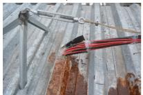
**Mounting and installation quality** – Every solar PV panel comes with manufacturer guidelines on the placement and mounting of panels, and their interconnection. Incompliance and self-installation make the PV plant susceptible to strong winds, and heavy snowfall. Damage to the panels or your rooftop can make the installation unsalvageable.
